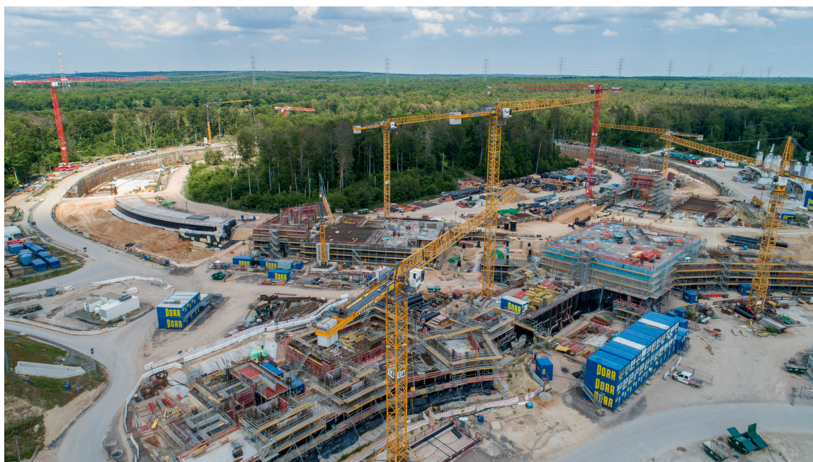
Figure 4.2.: Photograph of the FAIRconstruction site taken in 2021. Source: [49].
